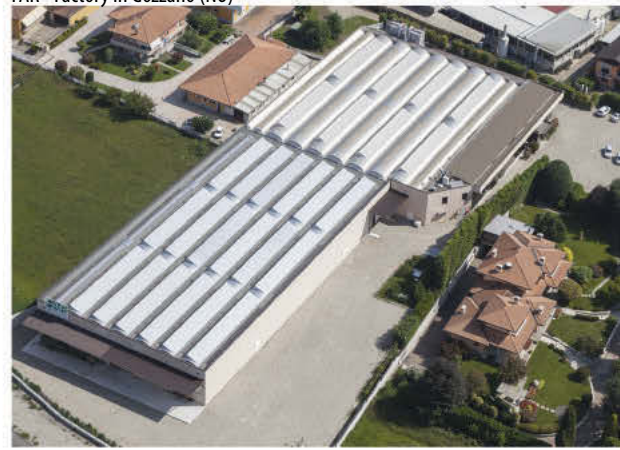
FAR - New factory in Gozzano (NO)
